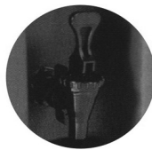
Wasserhahn in Hohlraum
